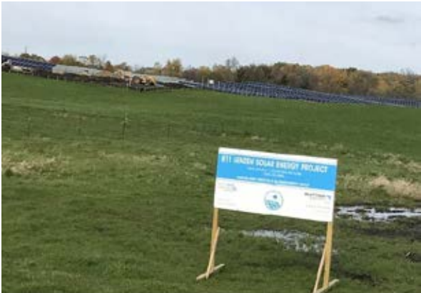
Watertown, Minnesota, USA Solar Garden
